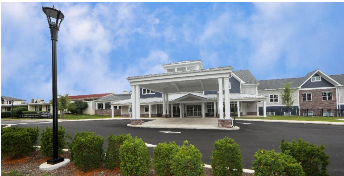
Pickering Manor Yates Pavilion Main Entrance
